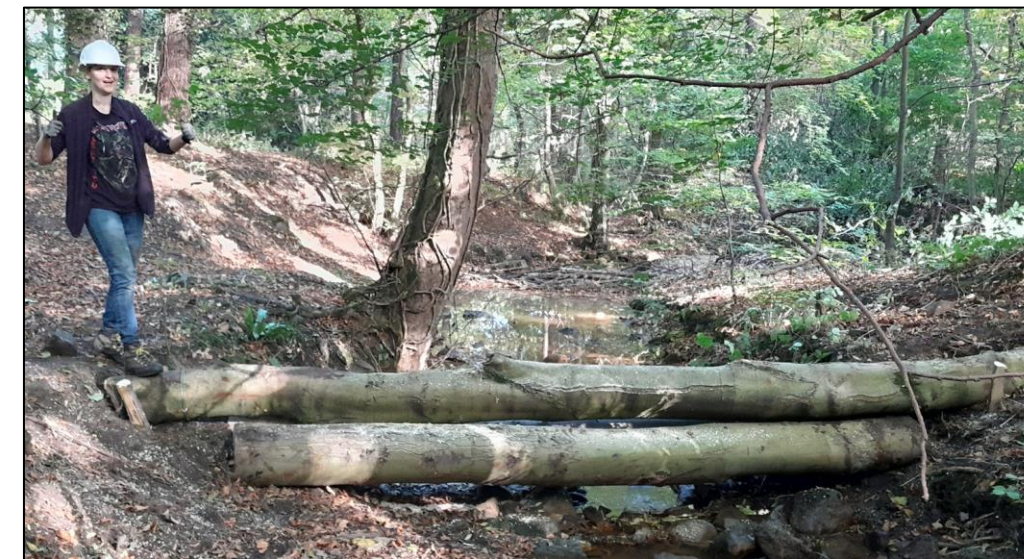
Leaky dams in Limb Brook © Rob Jones
